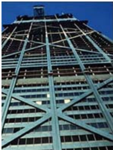
Left: Exterior lateral bracing created open interior spaces at the John Hancock Building—Chicago, IL
